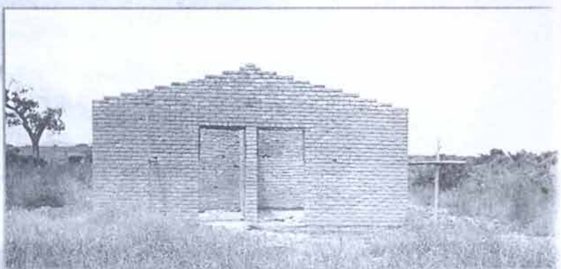
▼ Guardian shelter at Mzuzu Central Hospital
